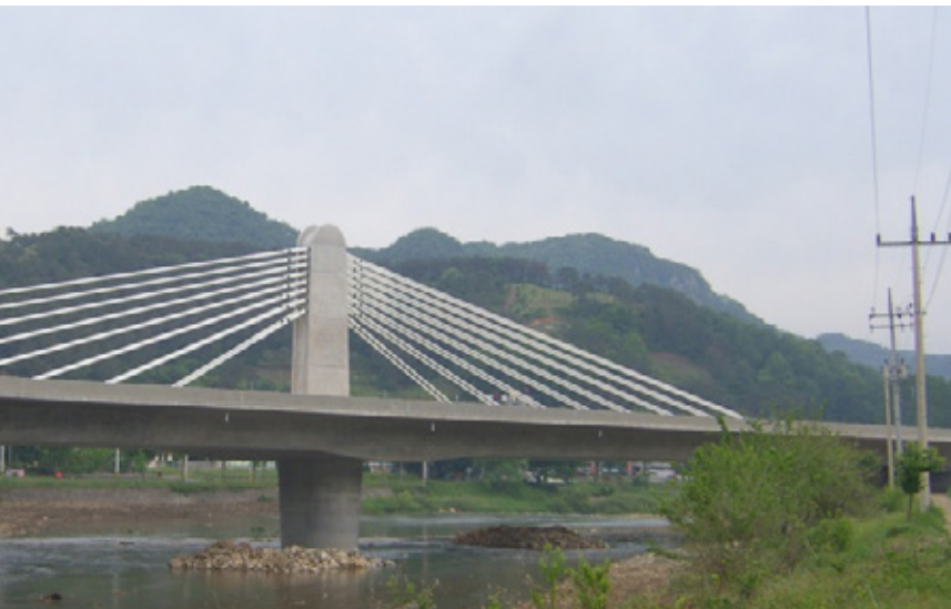
Sungai Muar Bridge Malaysia Span: 132 m
