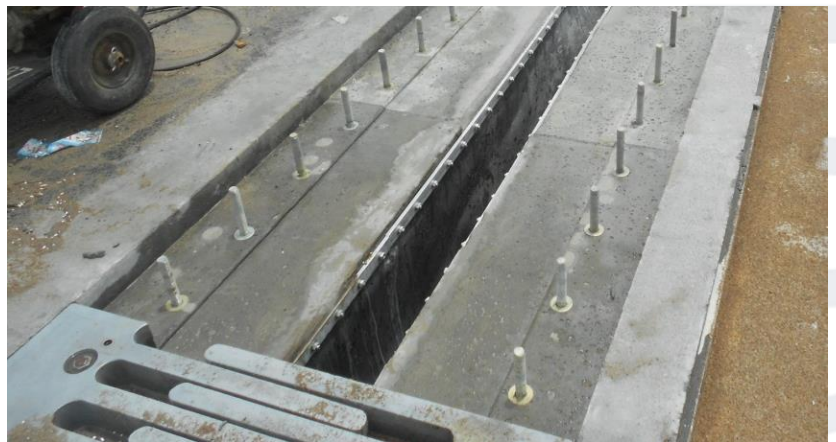
Details of the elastomeric membrane
