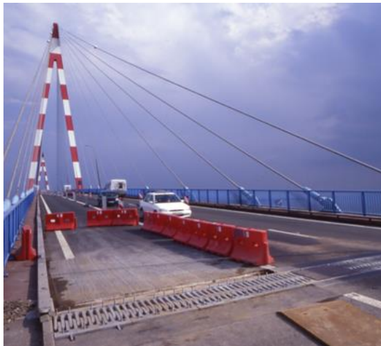
WP 500 under installation 1/2 carriage way (Saint-Nazaire Bridge France)
