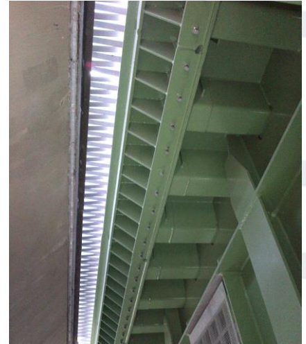
WP550 connected to an orthotropic deck, Szébény (Hungary)
