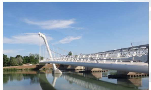
Decines Bridge, France
