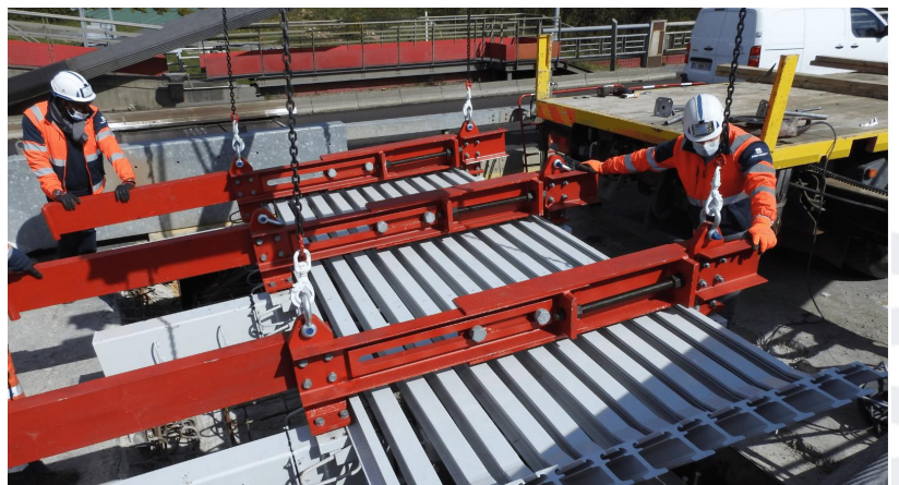
Installation of LW960 on Tancarville bridge (France)
