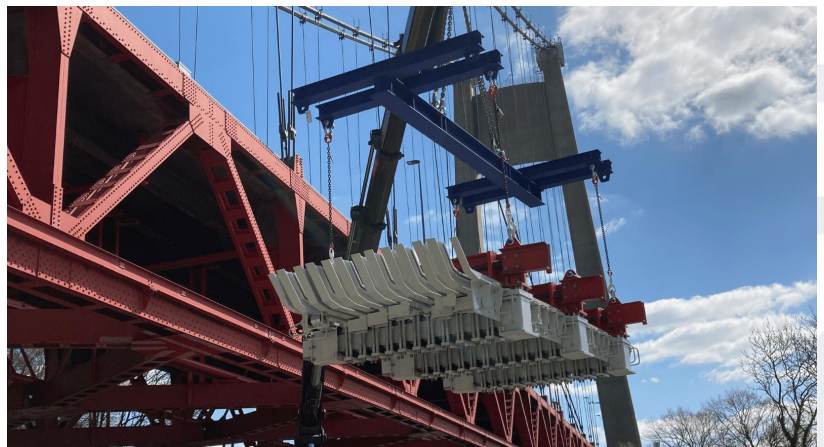
Installation of LW960 on Tancarville bridge (France)
