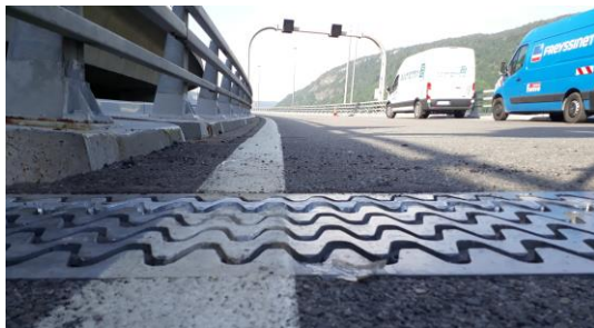
Close-up view of noise reduction system on Nantua Bridge A40 Highway (France)
